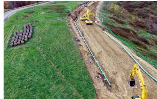
Pipeline under construction
