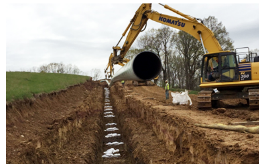
Ditch Dug by GPS Guided Excavator
