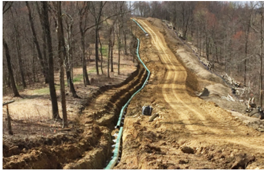
Pipe Laid In Trench
